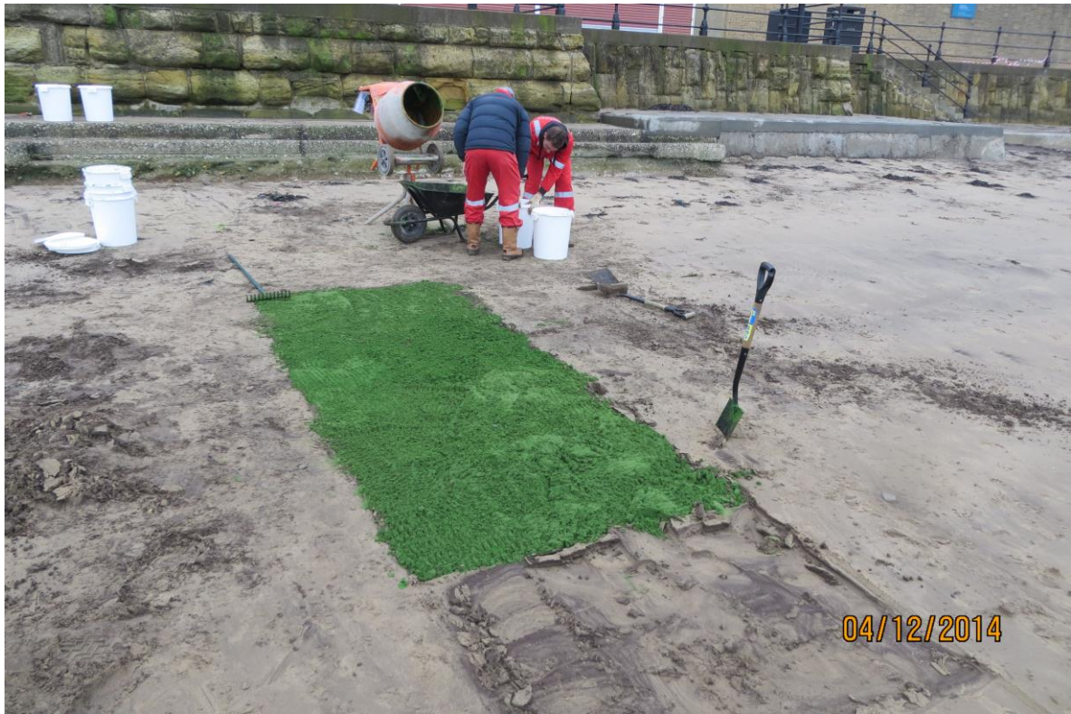
Figure 5. Deployment of the Tracer Material at Deployment Zone 2
